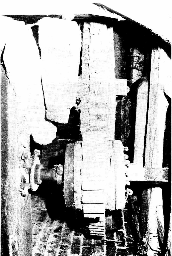
Long Compton Mill (156) - the wooden spur wheel and Stone nut
